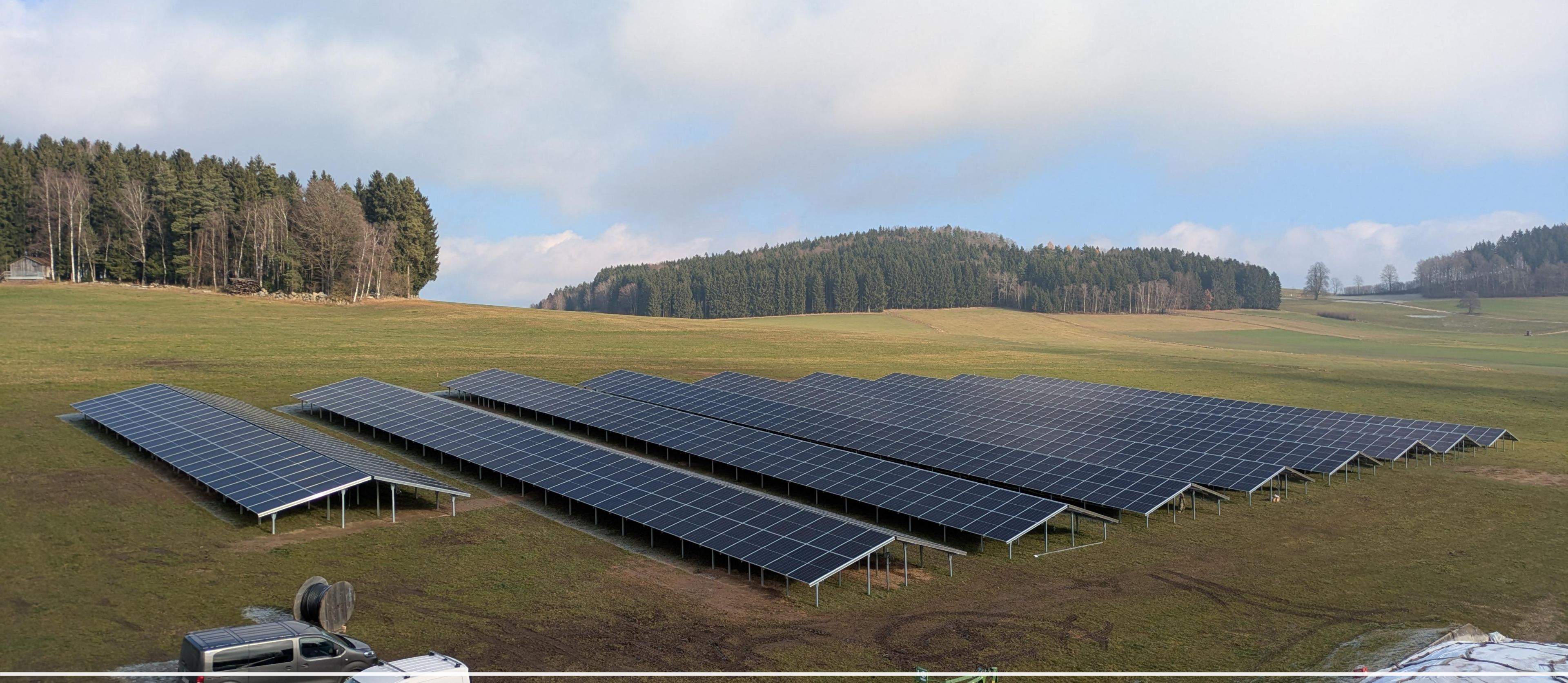
AGRI PV ANLAGE - Rainbach 999kWp
